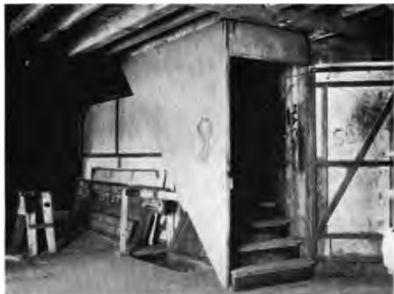
Fig. 4. Hinged Stairway Enclosure, lowered.
